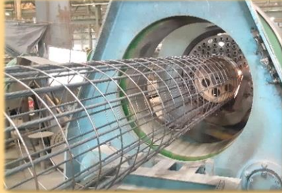
點焊鋼筋籠 (Cage forming)
