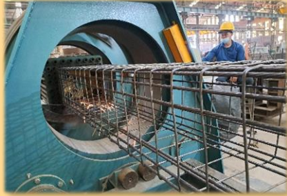
點焊鋼筋籠 (Cage forming)
